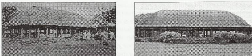
Figure 10ab: The Leoso guesthouse in Leone, Tutuila in 1930 and 2004. The only things that have been changed are the roofing material and the outer posts, which are now cement Source: American Sāmoa Historic Preservation Office.
