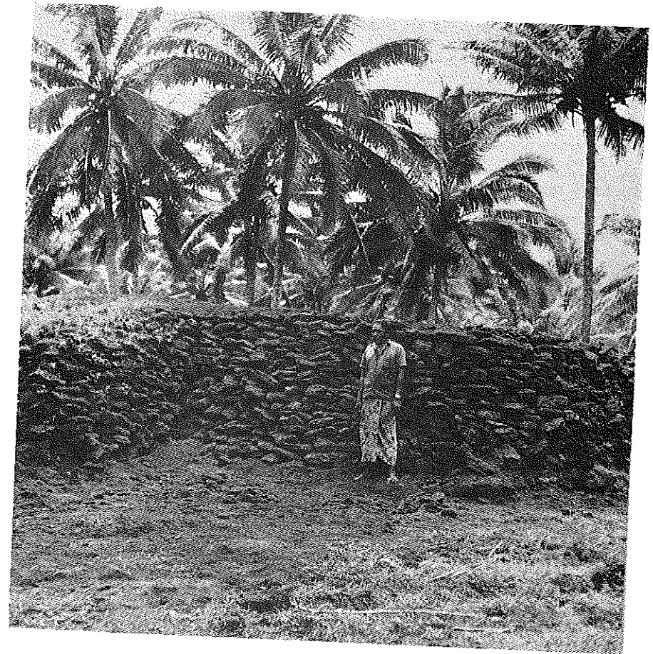
Fig. 7 (cont'd). Top, slump where test cut was made. Bottom, as restored.
